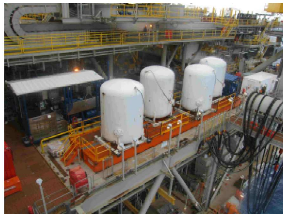
DECK PANELS INSTALLED OFFSHORE FOR BULK TANK INSTALLATION
